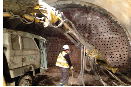
(e) Shotcrete 타설
