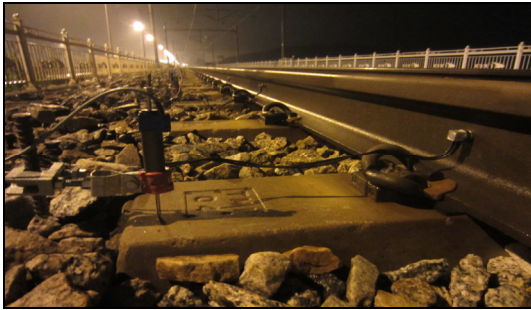
(a) Sleeper displacement measuring
