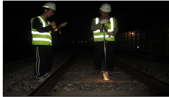
(b) Track support stiffness measuring(LFWD)
