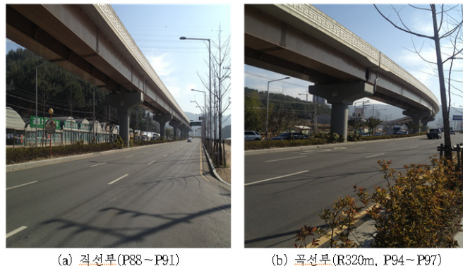
Fig. 1 Field-test site (Gochon~Anpyeong in Line 4, Busan)
