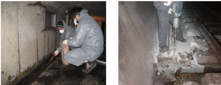
Fig.3 Sludge Cleaning & Expansion Drainage
