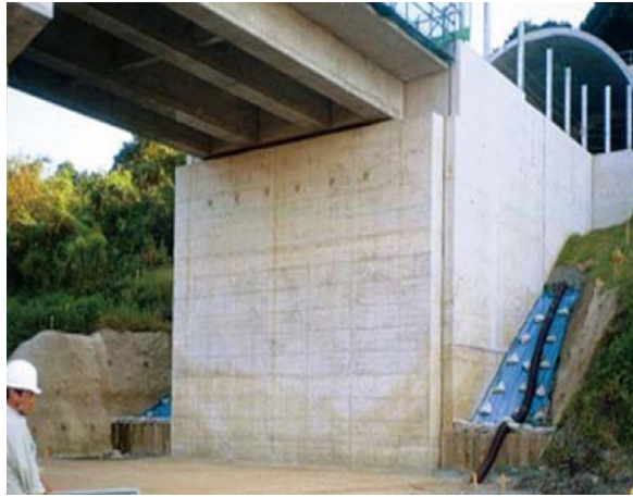
Fig. 2 Application of geosynthetic-reinforced abutment (Kyushu shinkansen)
