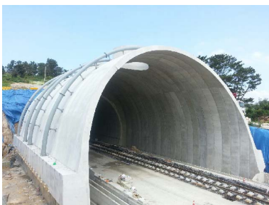
Fig.1 Hood at Woosan tunnel
