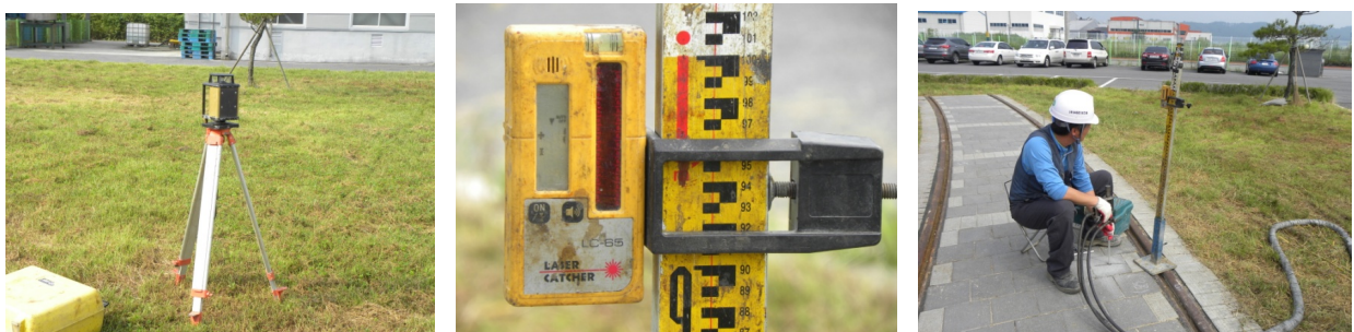
Fig. 4 Level measurement using laser sensor during injection
