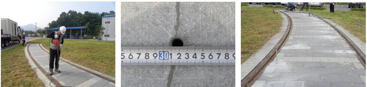
Fig. 3 Installation of injection tube
