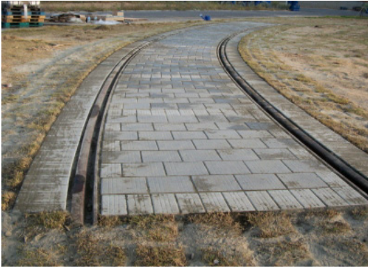
Fig. 1 Embedded rail track for settlement restoration test
