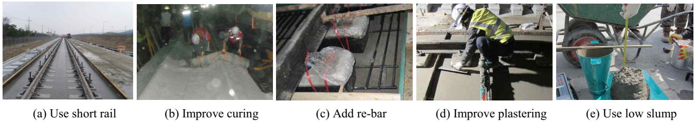
Fig.2 Method of track concrete crack reduction
