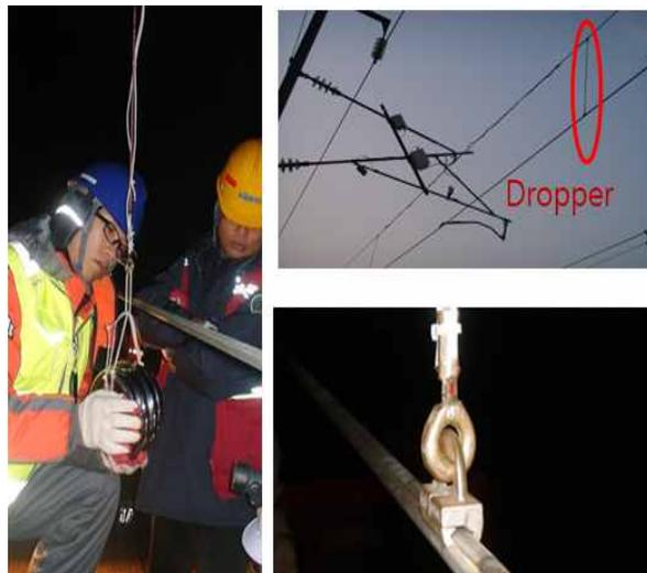
Figure 3 Installation and Calibration of a Loadcell for Dynamic forces on the Dropper nearest to the Mast Registered as 123-21 Located in YeonJe Bridge
